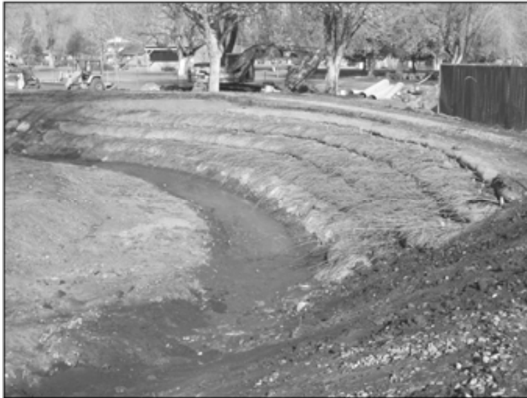
Vegetated soil lifts
