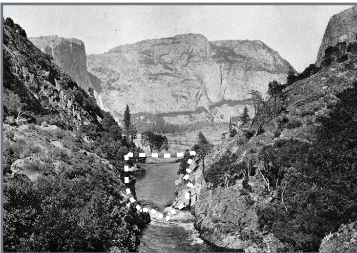
The narrow gap was an enticing place to build a dam, but water would not reach San Francisco for 21 years.
